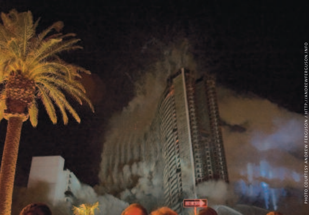
Both Stardust towers crumbled into their own footprints as gravity took over, above. The rubble left in the aftermath of an implosion can take months to clean up, left.
